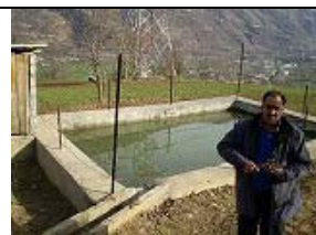
Pump Outlet Tank
