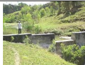
Existing Check Dam
