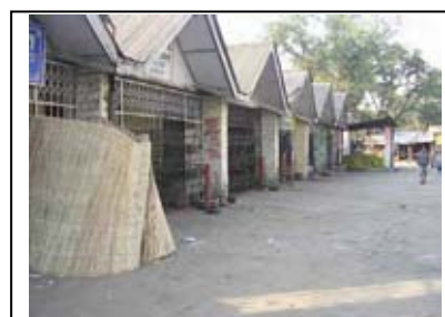
Front View Nagrota Bagwan Market Yard
