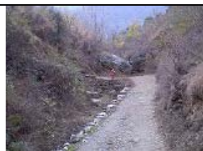
Existing Farm Road
