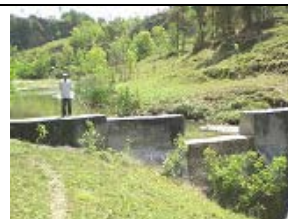
Existing Check Dam
