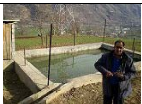
Pump Outlet Tank
