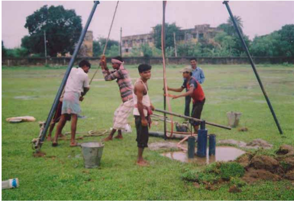
Photograph of field Boring of Bore Hole – 07 in field
