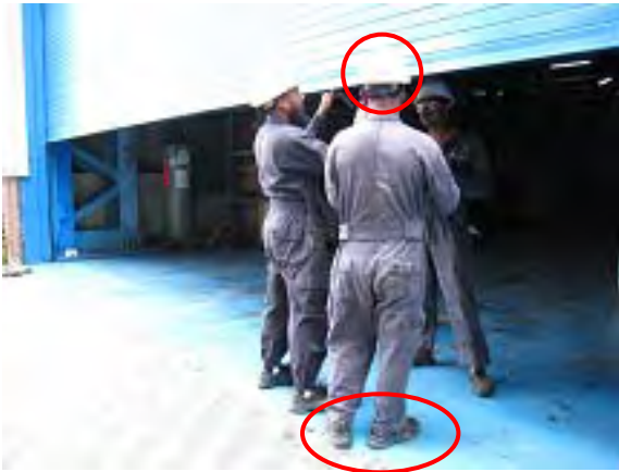
Thoroughly instructed to wear safety equipment (uniform, helmet, protective goggle and safety shoes)
