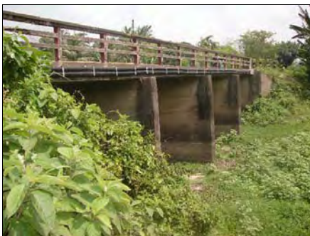
Photograph I-4-8-9 RCC Bridge at 157km from Mongla Port
