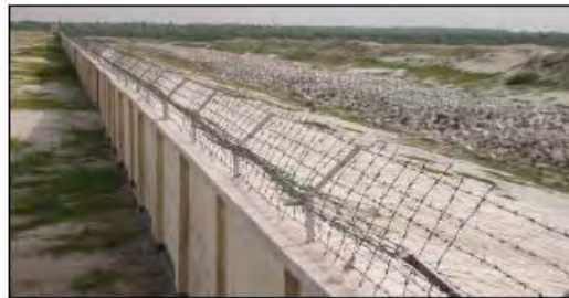
Photograph I-4-8-4 Excavated canal outside south boundary wall
