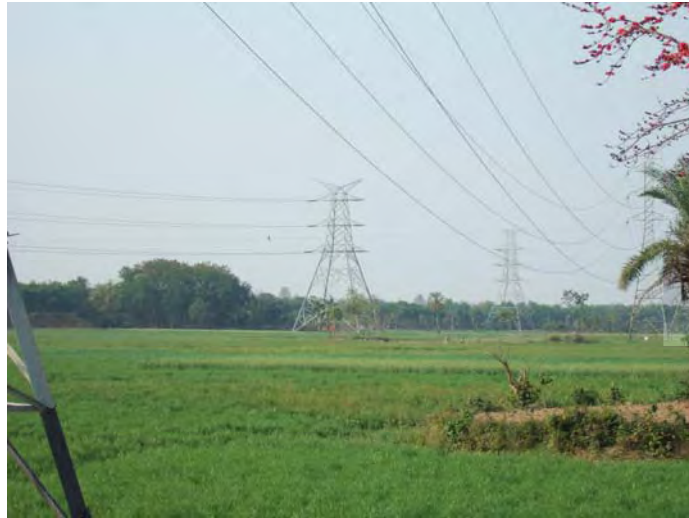
Figure I-4-4-4 Situation around Bheramara substation
