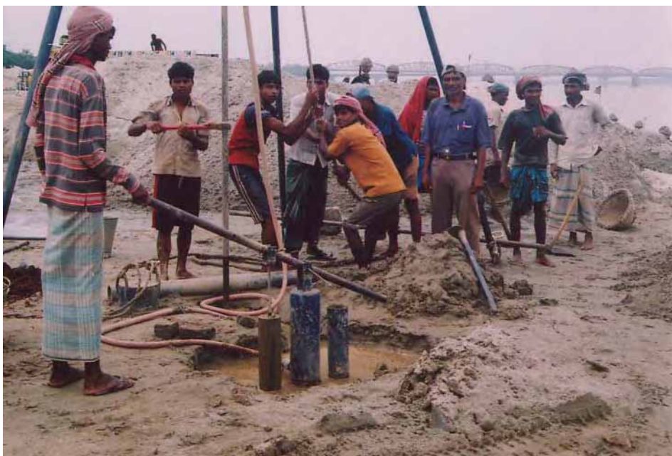
Photograph of field Boring of Bore Hole – 09 in field
