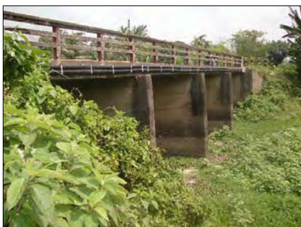
Photograph I-4-8-9 RCC Bidge at 157km from Mongla Port
