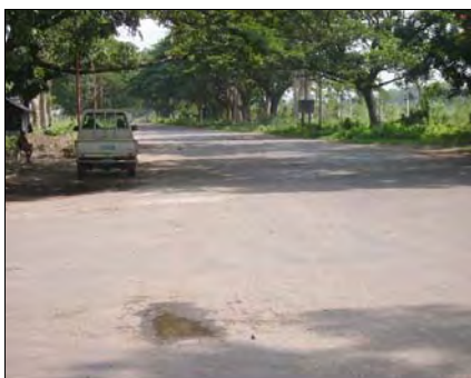
Photograph I-4-8-7 Mongla Port Road
