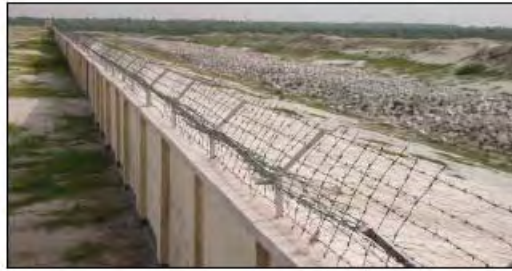
Photograph I-4-8-4 Excavated canal outside south boundary wall
