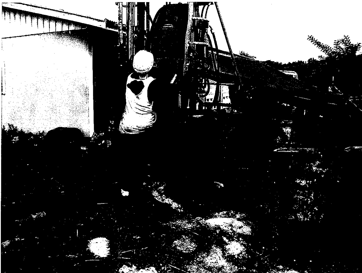
Plate 4.1: Drilling rig and Operator at Test Site
