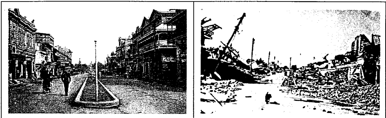
Bruce Street (Jinnah road) before the earthquake (左) immediately after the earthquake (右)
