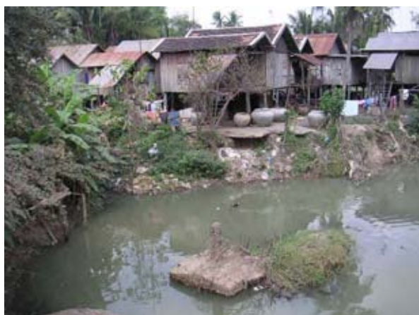
Existing Main Canal at the Beginning Point, Water Quality Problems due to Houses Standing along the Canal (Por Canal Rehabilitation Sub-Project) (February 8th 2008)
