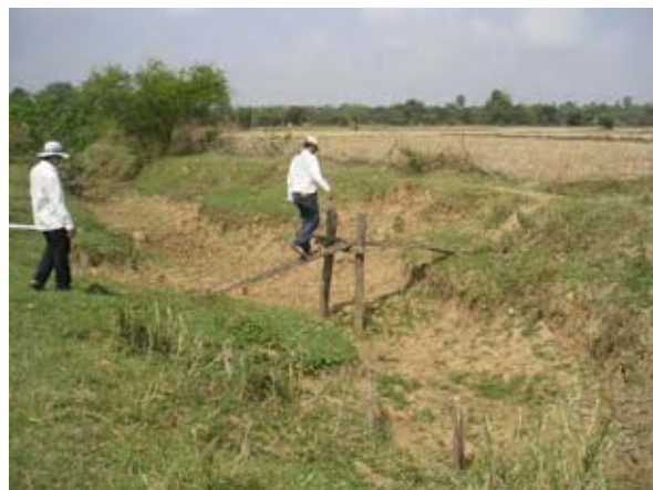
Existing Main Canal and Wooden Canal Crossing (Ream Kon Rehabilitation Sub-Project) (February 8th 2008)
