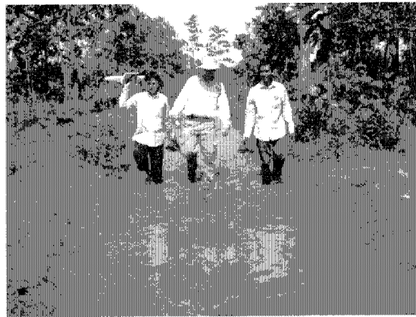
Poor Road Network in the Command Area particularly during the Wet Season (September 4 th 2008)
