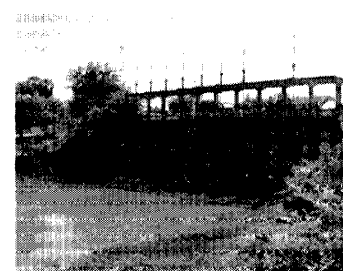
Existing Weir not Functioning (May 28 th , 2007)
