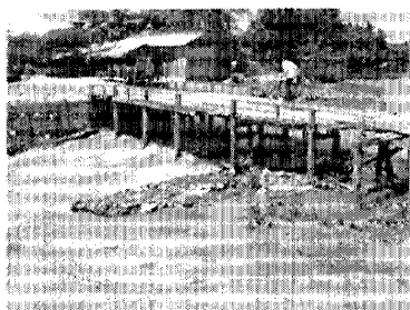
Gabion weir at new channel
