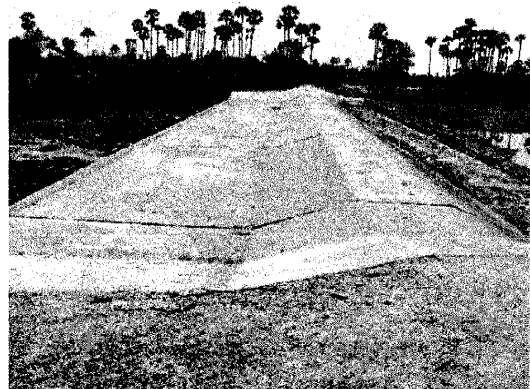
Construction of overflow type spillway
