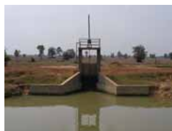
3. Inlet of Secondary Canal
