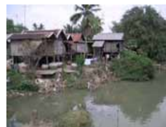
Houses Located along the Main Canal at Por Canal Rehabilitation Sub-Project (February 7 th , 2008)
