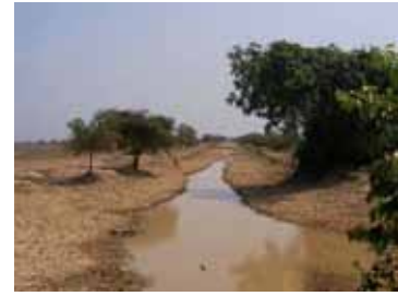
5. Main Canal: End Point before flows to Boeung Khnar River
