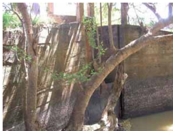
Existing Intake Structure (Por Canal Rehabilitation Sub-Project) (May 25th 2008)
