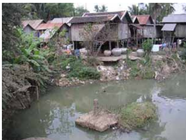
Existing Main Canal at the Beginning Point, Water Quality Problems due to Houses Standing along the Canal(Por Canal Rehabilitation Sub-Project) (February 8th 2008)
