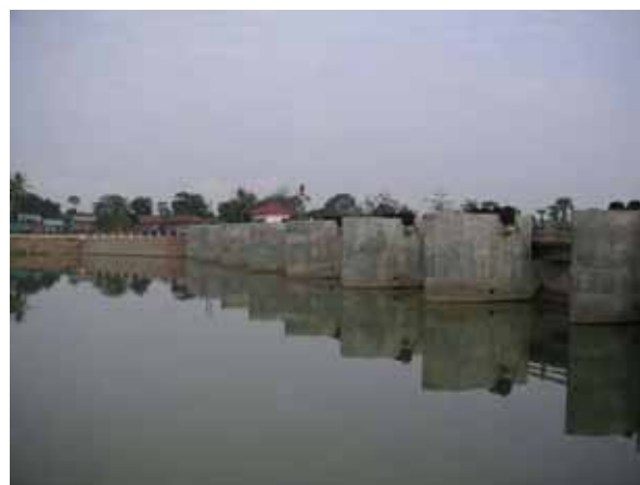
Existing Damanak Ampil Headworks Originally Constructed by MOWRAM in 2006 (Damanak Ampil Rehabilitation Sub-Project) (February 2nd 2008)
