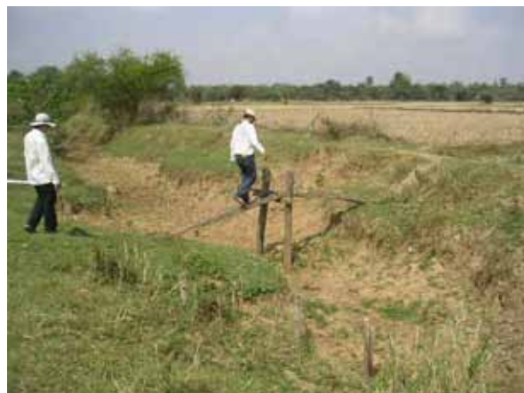
Existing Main Canal and Wooden Canal Crossing (Ream Kon Rehabilitation Sub-Project) (February 8th 2008)
