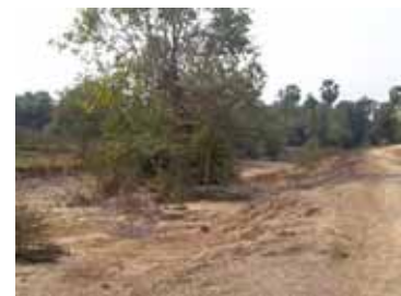
Main canal to Southeast (Wat Chre Rehabilitation Sub-Project)
