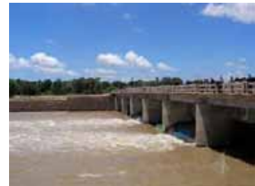
Damnak Ampil Headworks (Damnak Ampil Rehabilitation Sub-Project)
