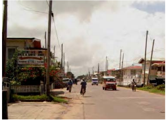
Close set area in the Project area. The existing distribution trunks run along both road shoulders.
