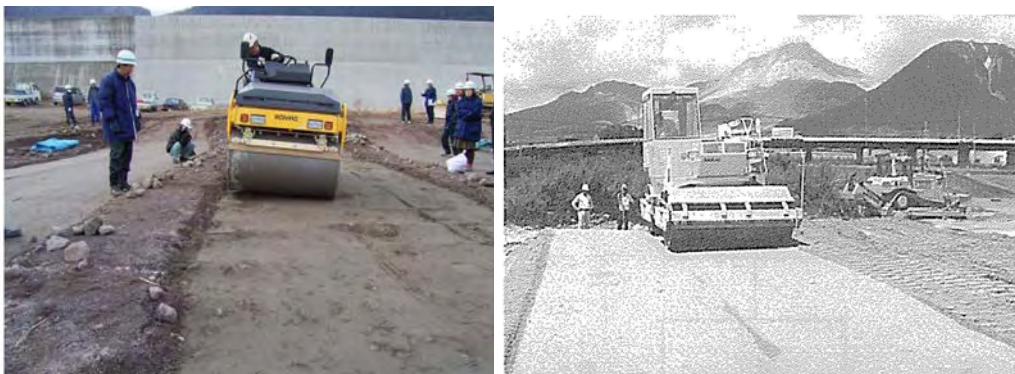
Compaction with vibrating roller (surface compaction)
