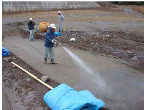
Cleaning and water sprinkling
