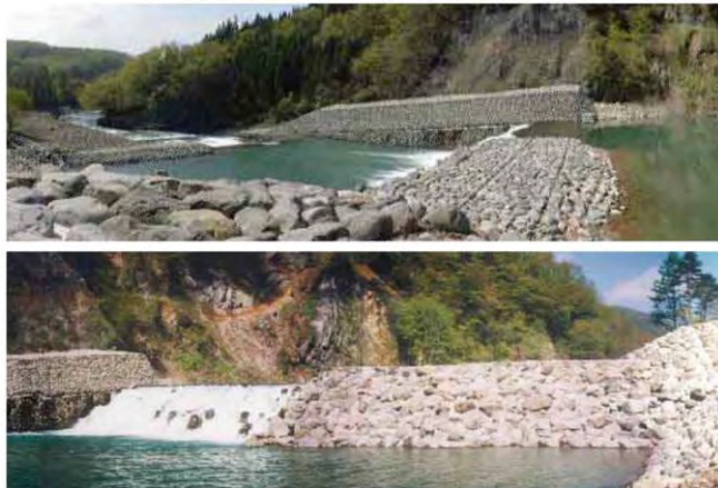
Figure 2.3.6 Sabo Dam of Sabo Soil Cement Covered by Riprap Work (Genbu Sabo dam, Iwate Prefecture, Japan)
