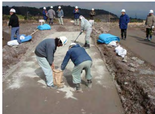
Dry cement sprinkling
