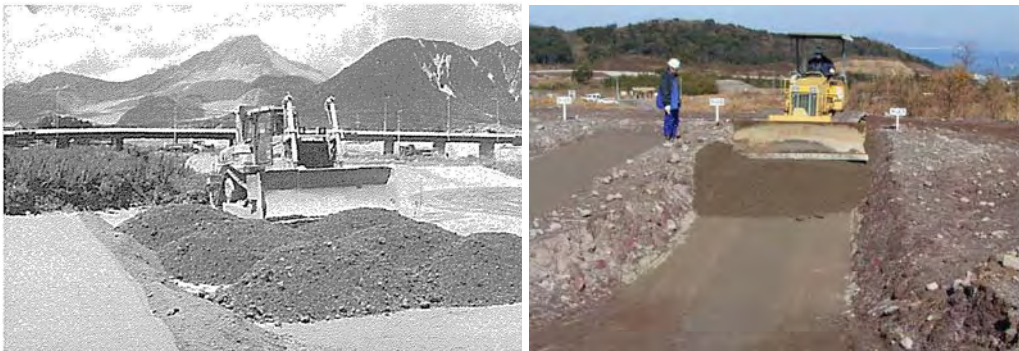
Screeding using bulldozer
