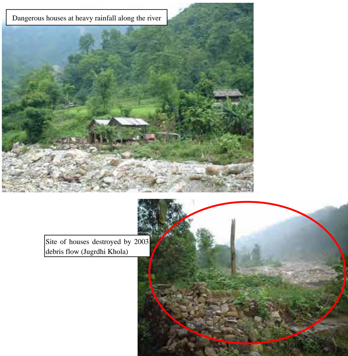
Figure 4.3.1 Dangerous area (along river/stream)
