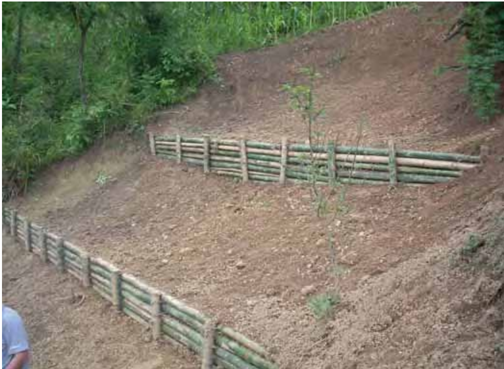
Figure 3.2.2 Wicker work implemented at 11km+500
