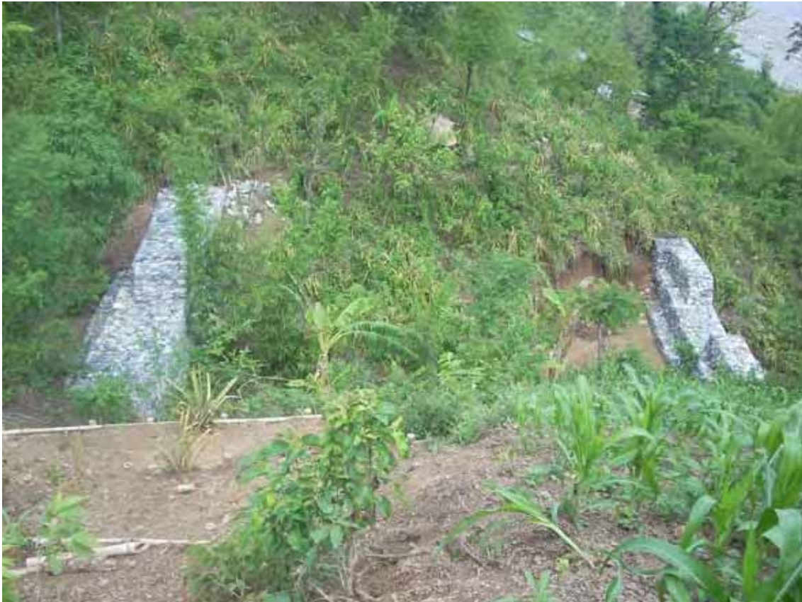
Figure 3.3 Bio-engineering work implemented around the Kabilas Village
