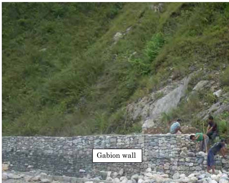
Figure 3.6 Gabion walls implemented around the M-N highway
