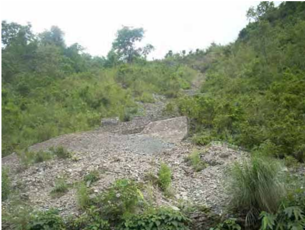
Figure 3.7 Gabion Sabo/Check dam constructed along the M-N
