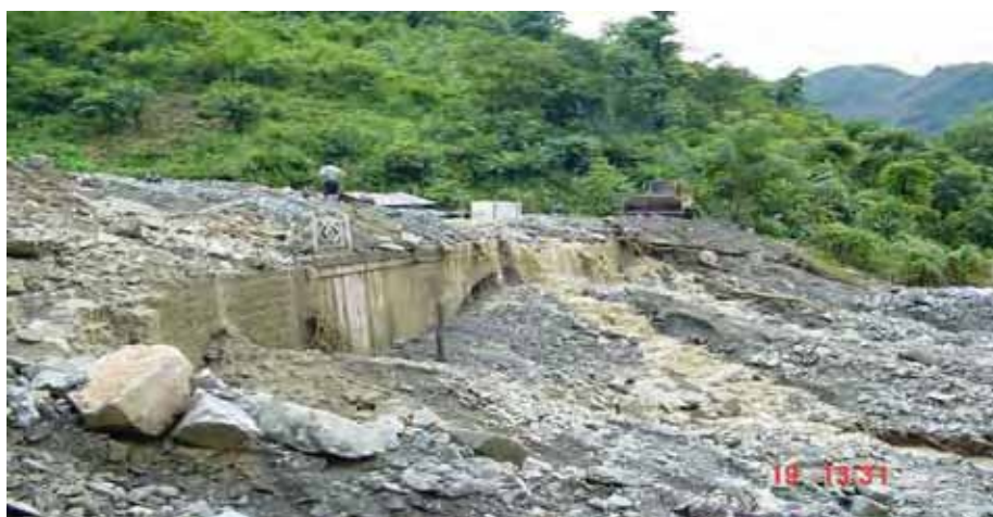
Figure 2.2.9 Buried Mohore Khola Bridge at km 21+500
