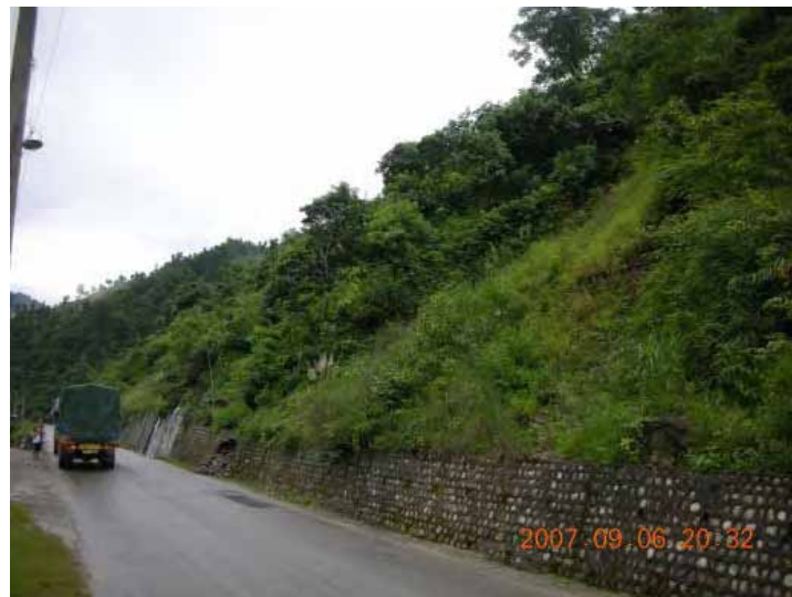
Figure 4.3.7 (b) Road side view of SL-3 slope
