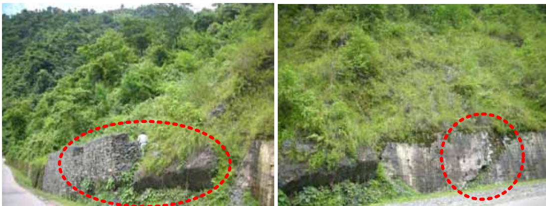
Figure 4.3.2 (a) Deformation of existing structures for countermeasure
