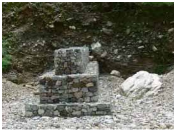
0+000m to 0+300m Left bank, Gabion Spurs 10 m length
