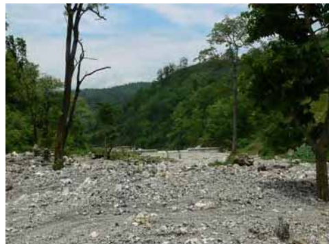
Sabo dams, 0+310m and 0+520m
