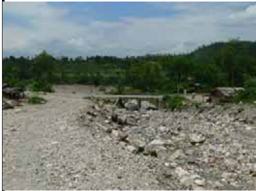
0+000m to 0+125m Canalization 125 m length
