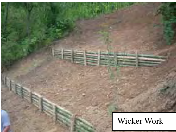
Working Situation of Simple Structural Measure (Wicker & Gabion work)
