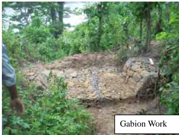
Working Situation of Simple Structural Measure (Wicker & Gabion work)
