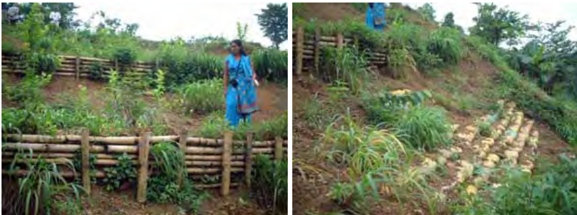
Figure 6.5.11 After Construction of Simple Slope Protection Work (August, 2008)
