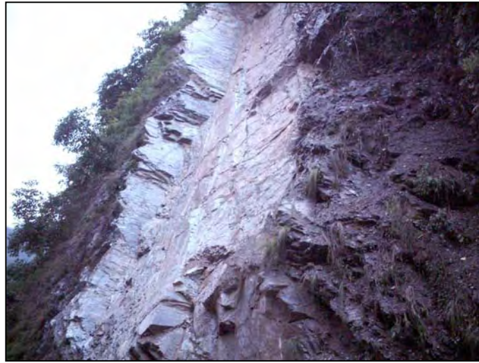
Figure 5.3.1 The Slope where rock mass failure occurred
