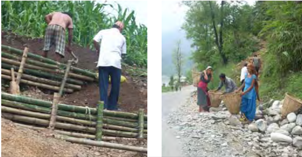
Working Situation of Simple Structural Measure (Wicker & Gabion work)
