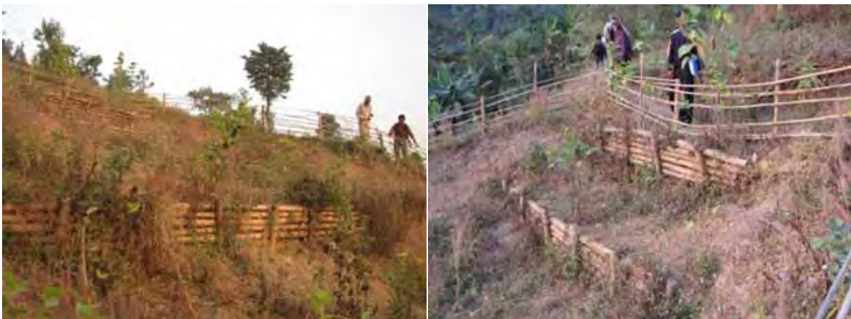
Figure 6.6.1 Situation of Simple Slope Protection Work (November 2008)
