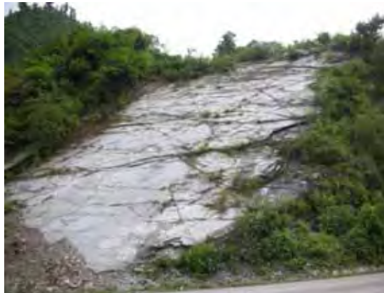
Figure 3.1.12 Typical Dip-slip Slope formed by Bedding-parallel slip of bedded rock (CH 25+500, near the Rigdi Khola)
