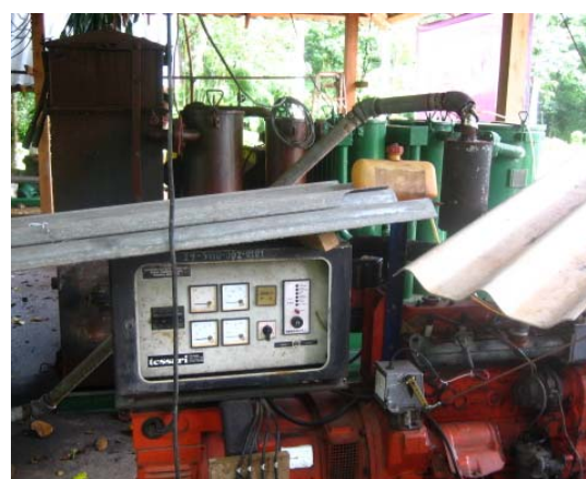
Gasification Facility (Red) and 15kW Gas Engine (Green)
