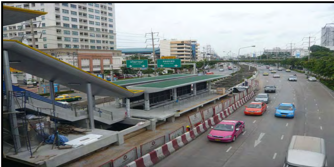
Figure 6.14 Construction Progress of BRT (Chongnonsri-Ratchpruk) (2)
