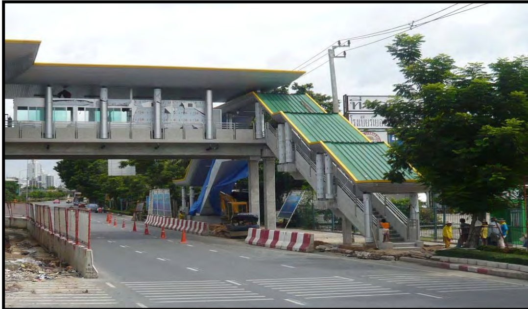
Figure 6.13 Construction Progress of BRT (Chongnonsri-Ratchpruk) (1)
