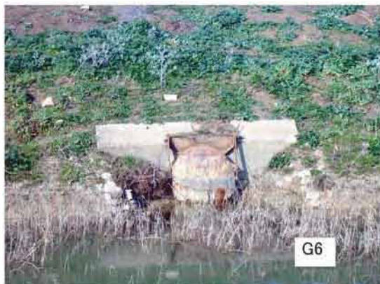
Figure 8.3.2 Present Conditions of Sluiceways along El Mabtouh Canal
