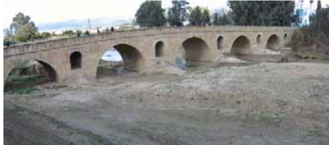
Historical Andalous bridge in Mejez El Bab
