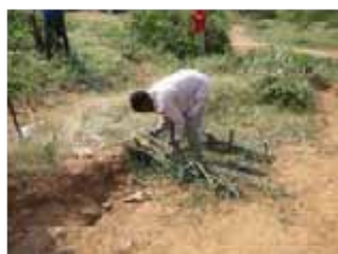
Works for preventing soil erosion by using grasses
