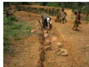
Water energy dissipater by using rock/stones
