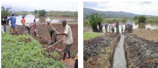
Construction of small-scale canal (Gashagamariro, Kibungo Cell)
