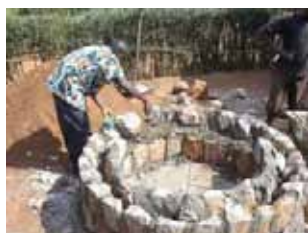
Trial to find out appropriate way for construction of the rainwater storage Left: Conventional method
