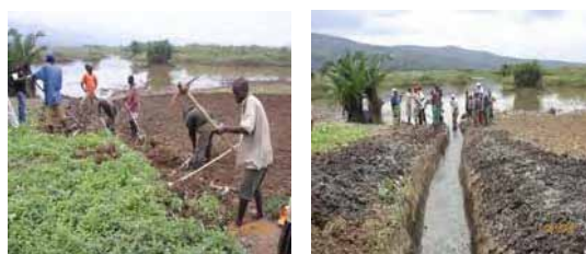
Construction of small-scale canal (Gashagamariro, Kibungo Cell)
