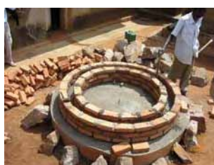
Trial to find out appropriate way for construction of the rainwater storage Left: Conventional method
