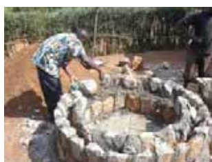
Trial to find out appropriate way for construction of the rainwater storage Left: Conventional method
