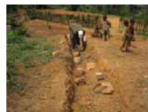
Water energy dissipater by using rock/stones
