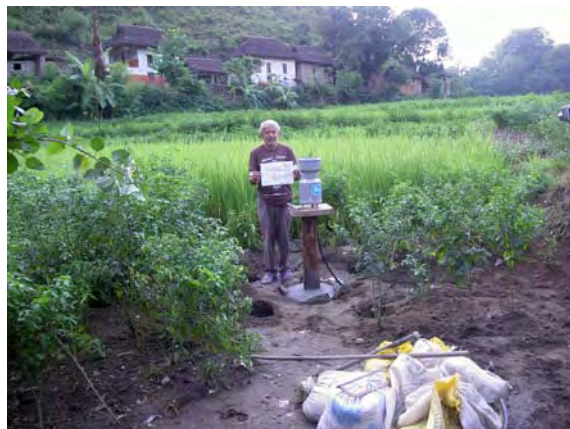
Installation completion of the rain gauge 2
