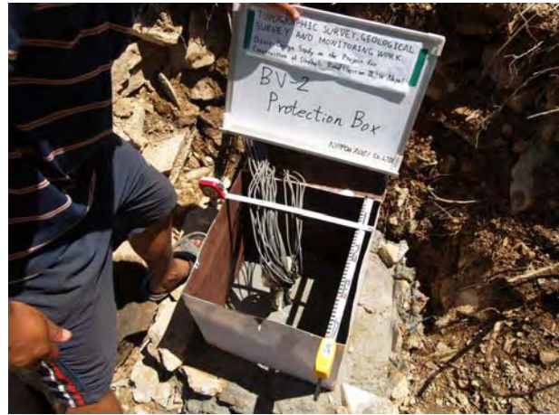
BV-2 . Installation completion of the protection box
