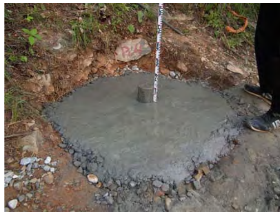
Installation completion of the movement pile
