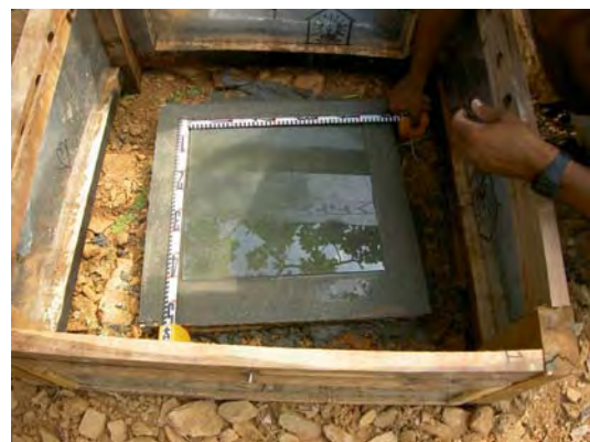
Photo 6-6-4 Installation situation of the concrete basic stand
