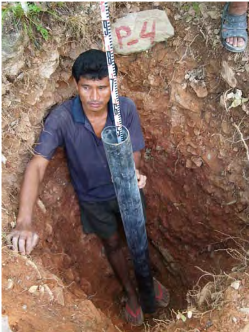
Basic digging situation
