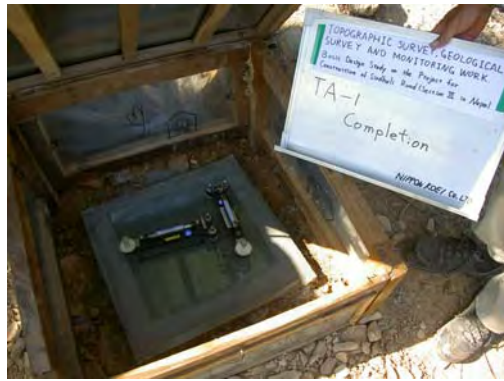
Photo 6-6-5 Installation completion of the ground clinometers
