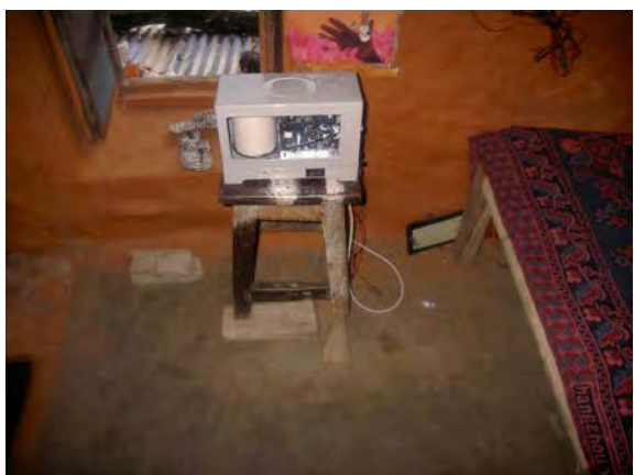
Installation completion of the rain gauge 3
