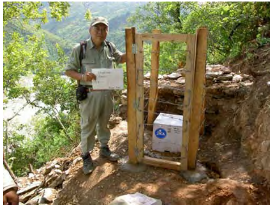
Example of BV-1 fence installation
