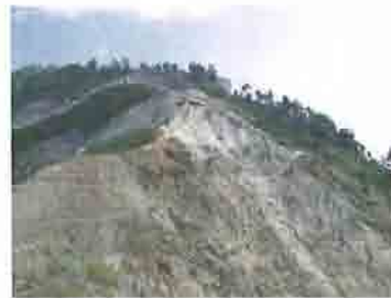
STA18 Failure of Weathering Rock
