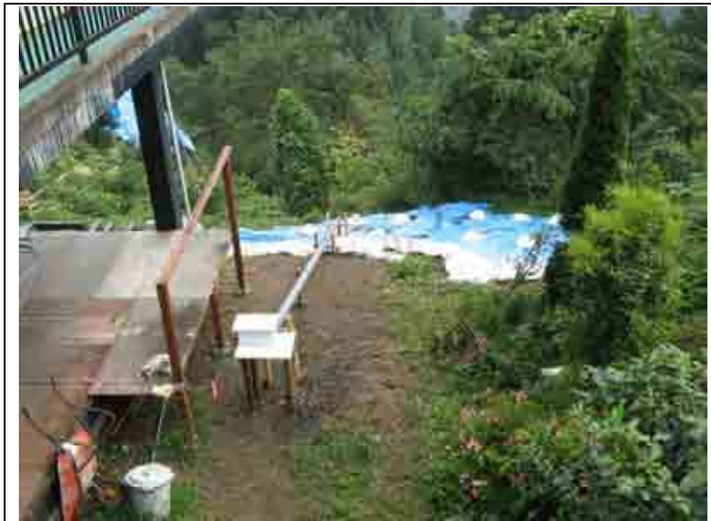
Picture. Setting of extensometer
