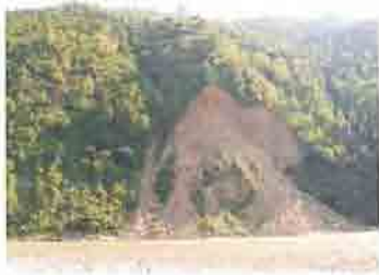
Collapse of landslide foot(2)
