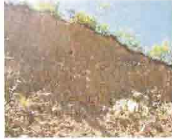
Materials of collapse surface
