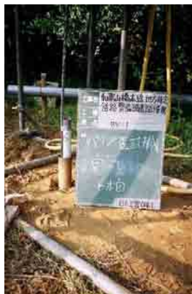
Picture3.1 Process of setting the pipe strain gauge
