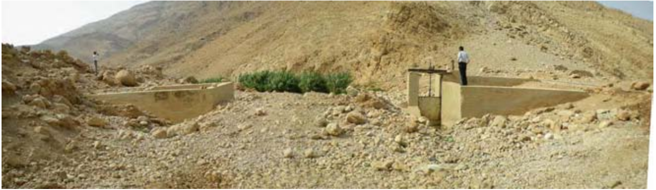
Ph-A5 Intake weir from downstream
