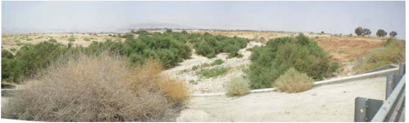
Ph-Q20 Upstream view from the cross point with the R90
