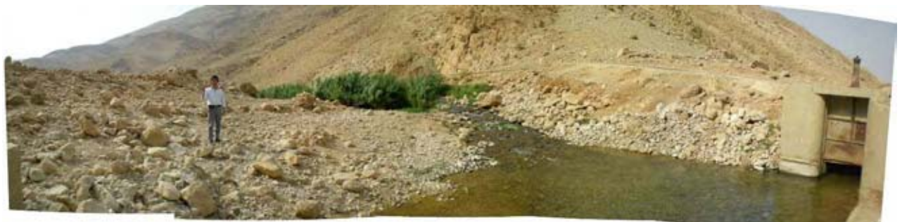
Ph-A4 at the point of the intake weir
