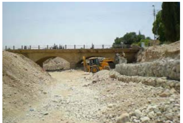
Ph-Q15 Upstream area of the road bridge
