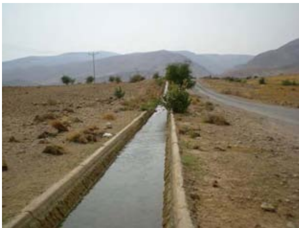
Ph-A7, A8 Headrace after mountain area
