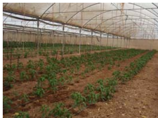
Drip irrigation system in greenhouse
