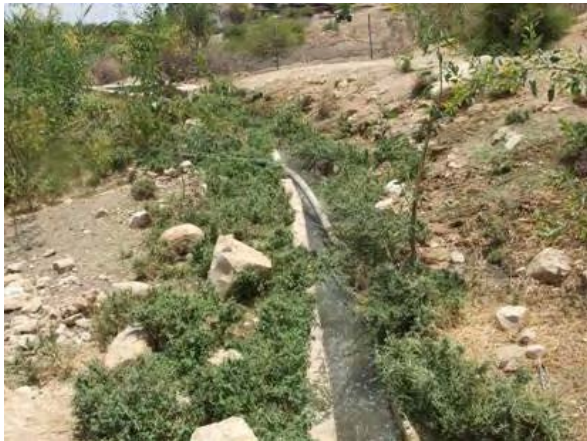
Before Improvement of Open Canal (Al Nwai'mah Spring)
