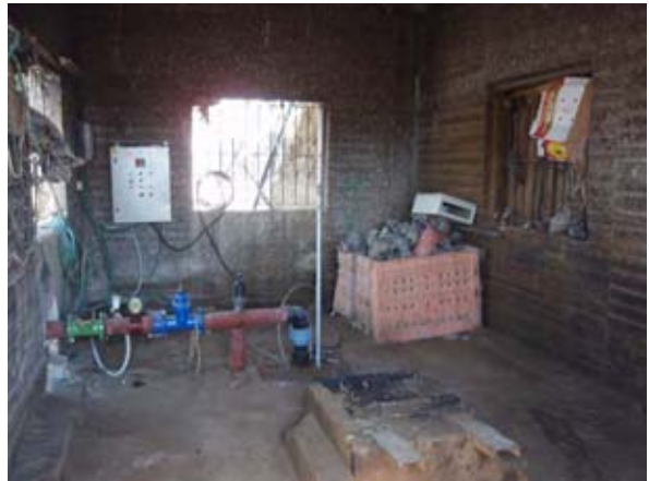
After Rehabilitation (19-17/054, Jiftlik)
