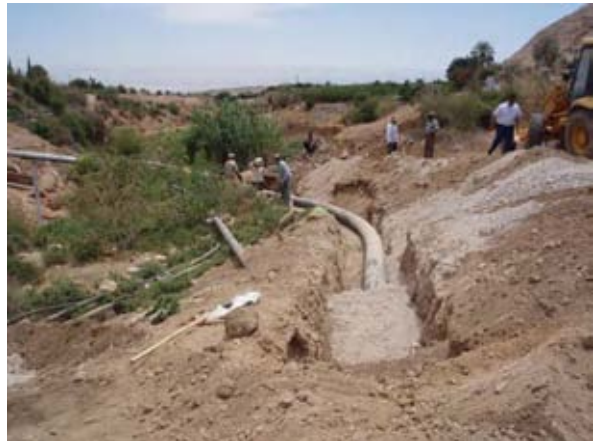
Under Construction of Pipeline (Al Nwai'mah Spring)
