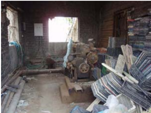
Before Rehabilitation (19-17/054, Jiftlik)
