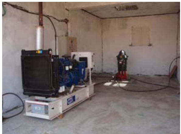
After Rehabilitation (19-17/055, Jiftlik)
