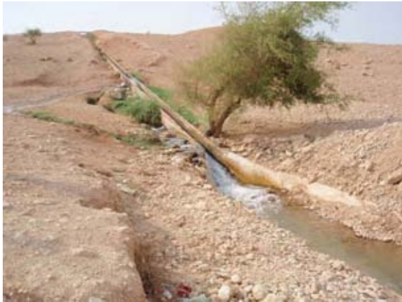
Leakage from Open Canal (Al 'Auja Spring)
