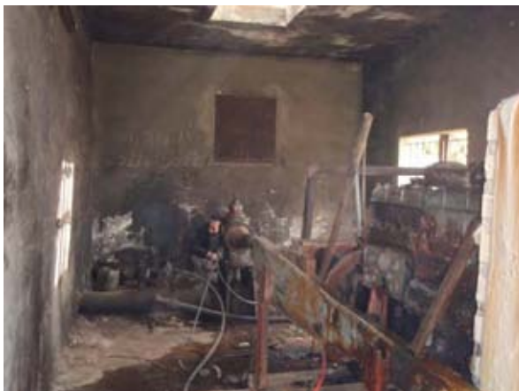
Before Rehabilitation (19-17/055, Jiftlik)
