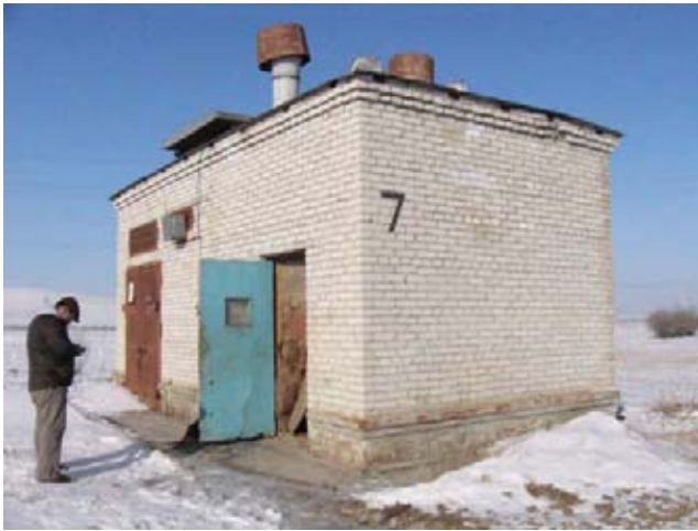
Pump House of 1st Station (1)
