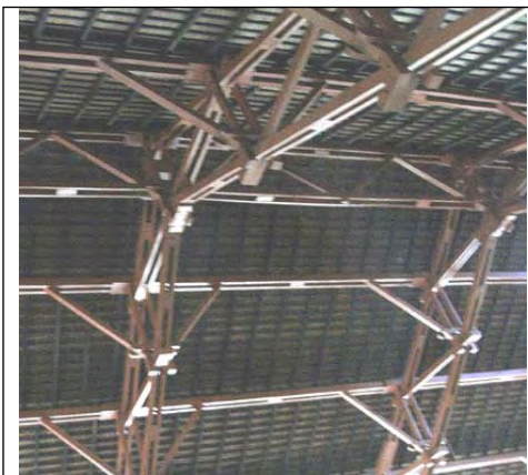
The woodwork of Hydraulic Building
