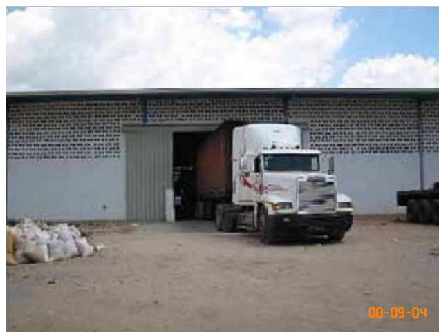
Warehouse for grains on Route 8 in Nacala-Porto
