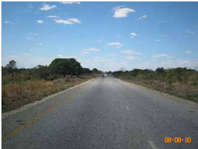
Nampula–Nacala Route 8: Pavement in good condition
