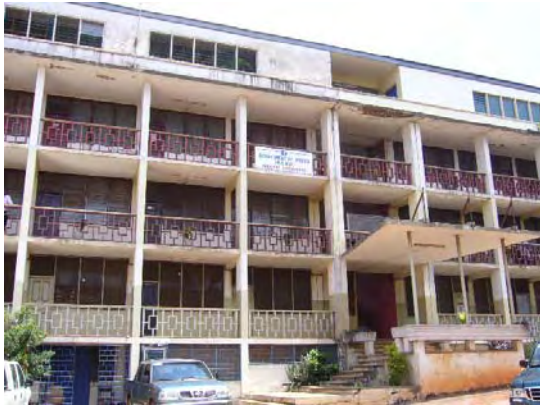
Project Office (TED)
