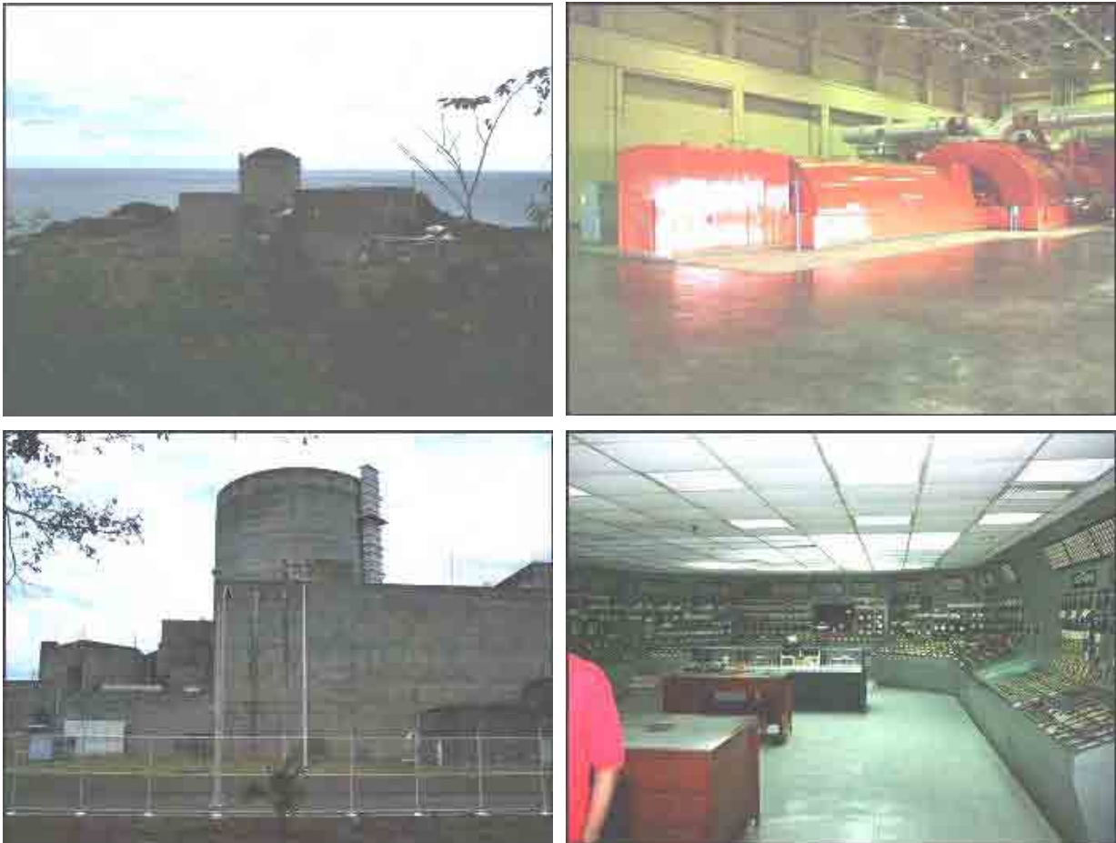
Figure 5.3-4 Nuclear Reactor in Bataan
