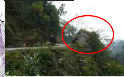
Open-cut rock on the left bank. The abutments will be installed after cutting the rock.
