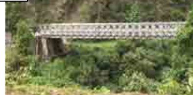
There is a steep slope at the back and sharp valley below the bridge.
