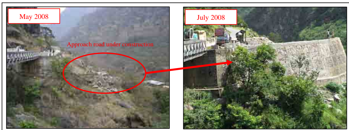
Fig. 2-10 Construction at Punatsangchu Dam and Approach Road
