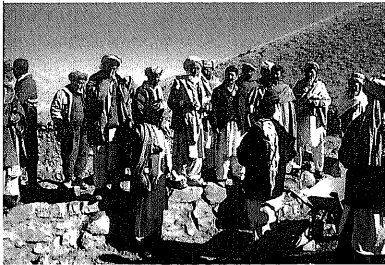
Visiting a construction site for an irrigation facility being built under a rural development assistance project. (Northern Bamiyan, Afghanistan)
