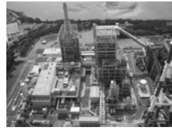
Demonstration Plant (250 MW) in Japan
