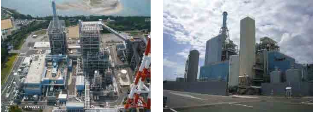
Fig. 5.1-2 Photos of IGCC Demonstration Plant in Japan
