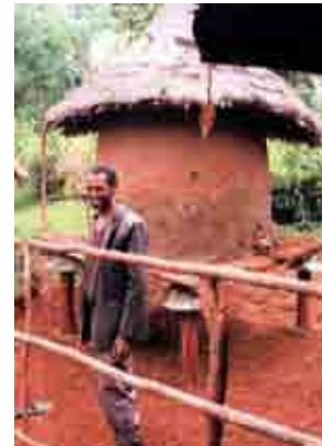
Store in East Africa: Floor height 50cm from ground level. Ensuring proper air flow.
