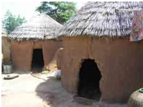
Local Grain Store, Tamale: It is difficult to control rain water and incoming small animals.
