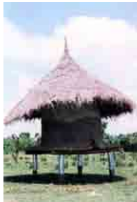
Store in East Africa: Floor height 50cm from ground level. Ensuring proper air flow.
