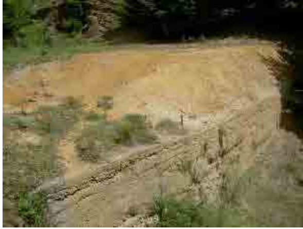
Photograph 2.22 Tailings Dam 1 (Kristov Dol Mine)
