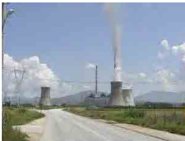
Photograph 2.25 Thermal Power Plant, REK Bitola
