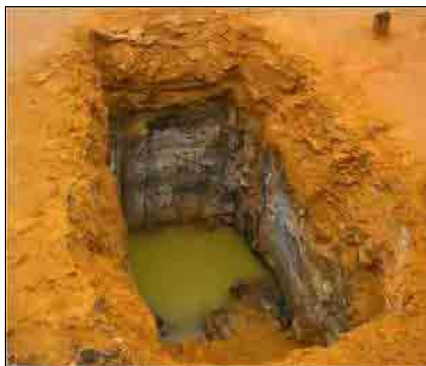
Photograph 2.12 Test Pit at Waste Dump Area in Lojane Mine
