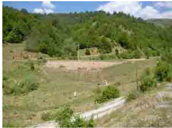
Photograph 2.23 Tailings Dam 2 (Krstov Dol Mine)
