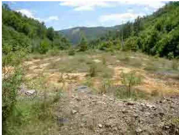
Photograph 2.24 Tailings Dam 3 (Krstov Dol Mine)
