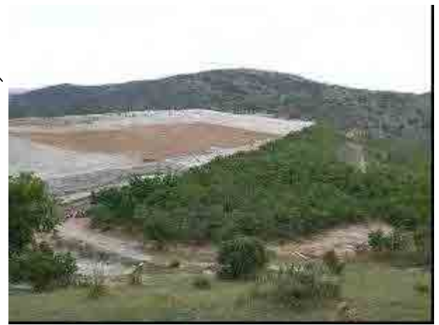
Photograph 2.8 Tailings Dam of Bucim Mine Covered by Top Soil
