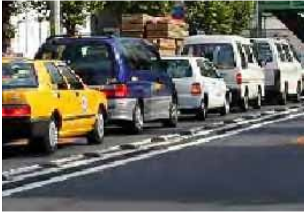
Picture 19.2-1 Example 1 of a Raised Median
