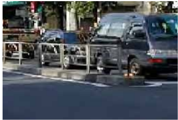
Picture 19.2-2 Example 2 of a Raised Median
