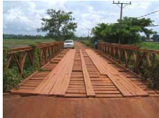
Typical Bailey Type Bridge
