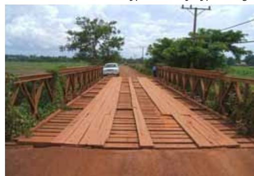
Typical Bailey Type Bridge
