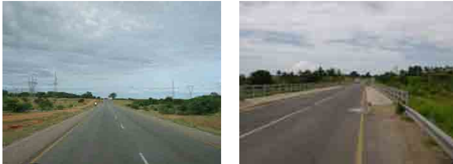
Figure 2.2.2 Improvement of New Bagamoyo Road
