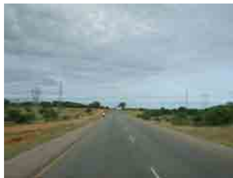
Figure 5.1.3 Road Surface Condition from Tegeta to Mpiji
