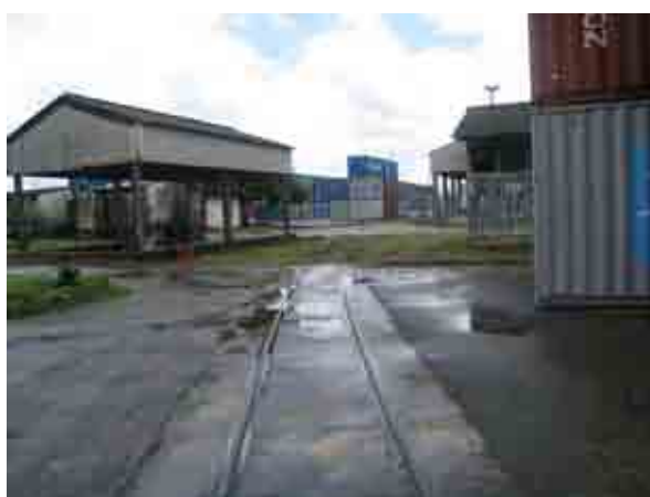
Figure 2.2.6 Ubungo Inland Container Depot
