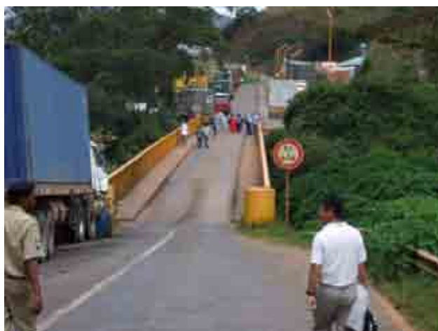
Figure 2.2.2 Rusumo Bridge (1-lane, with Load Limits)
