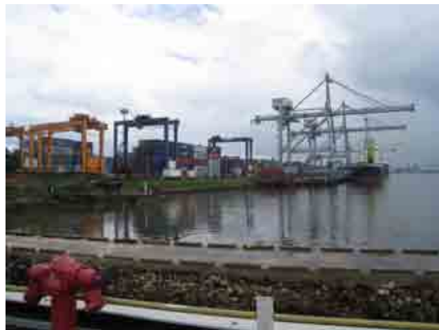
Figure 2.2.5 Container Terminal of Dar es Salaam Port
