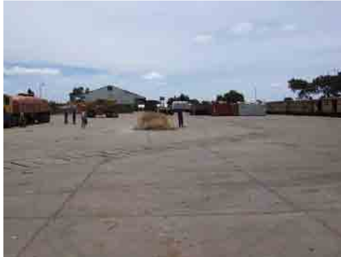
Figure 2.2.7 Isaka Dry Port
